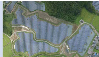
Chiba Prefecture Katori Power Station
