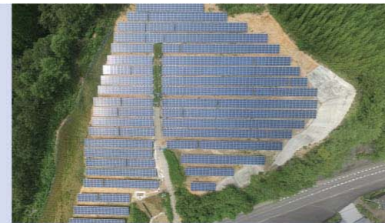
Oita Prefecture Saiki Power Station
