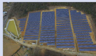
Gifu Prefecture Seki City Power Station
